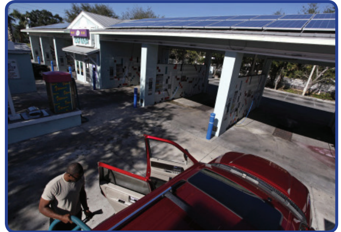
Mike Hall cleans his SUV at Sparkle Self Serve Car Wash on 34th Street S. The business got a $20,000 incentive from Progress Energy to install solar panels. The system will pay for itself in less than four years.
